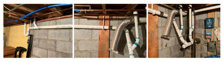
Drain, Waste, & Vent Systems: Material PVC
