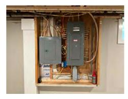
Branch Wiring Circuits, Breakers & Fuses: Branch Wire 15 and 20 AMP Copper
